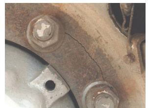
Examples of elongation of stud holes, wheel movement, wear to studs and a cracked wheel
